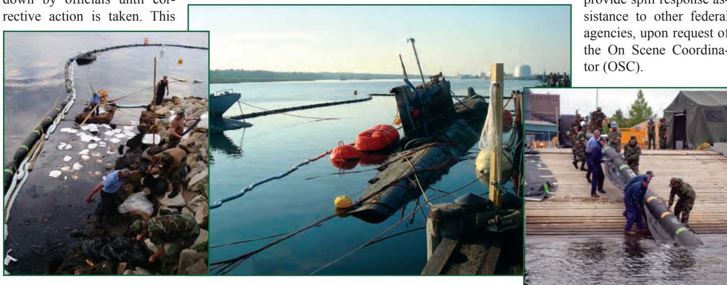
Pollution response efforts during the Juliett 484 submarine refloating operation in Providence, RI in 2008. Left: Rope mop and sorbent pads used to clean up the boomed-off oil. Right: Protective boom used to contain oil spilled from the submarine.
