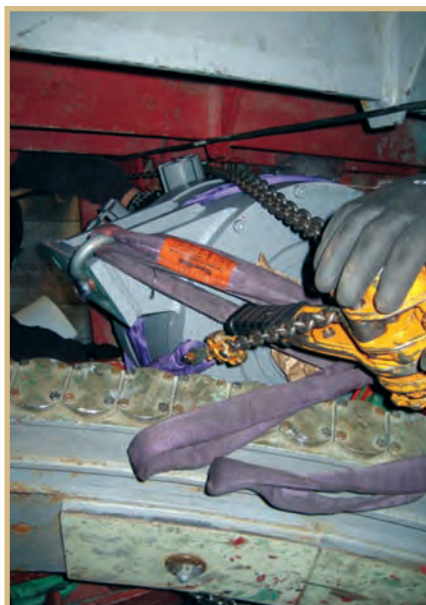
Right: The motor in drydock at Electric Boat, going through the grate. Left: The motor seen here with the bedplate obstruction.
